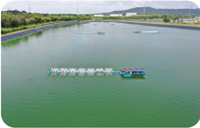
Solar-powered Surface Aerator at Pinthong Industrial Estate 5
