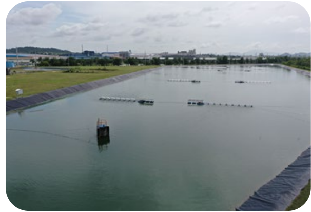
Solar-powered Surface Aerator at Pinthong Industrial Estate 5
