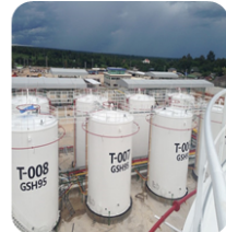
Storage Tanks with Cooling Rings
