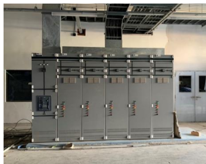
Installation of low-voltage electrical cabinet system (400 volts)
