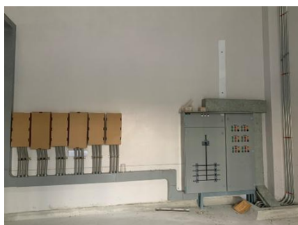
Installation of control cabinet for water pump system
