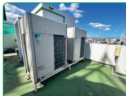
VRV air conditioning system
