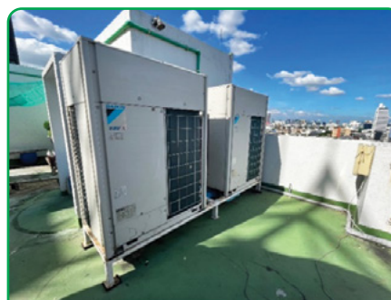
VRV air conditioning system
