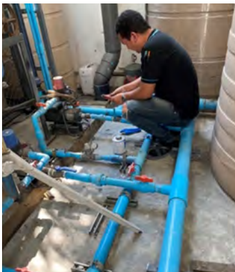
Survey to find leak water points
