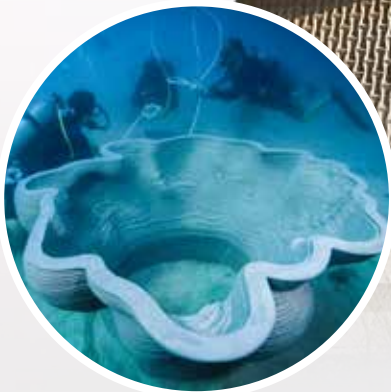
Coral Larvel Settlement made by 3D Cement Printing Technology
