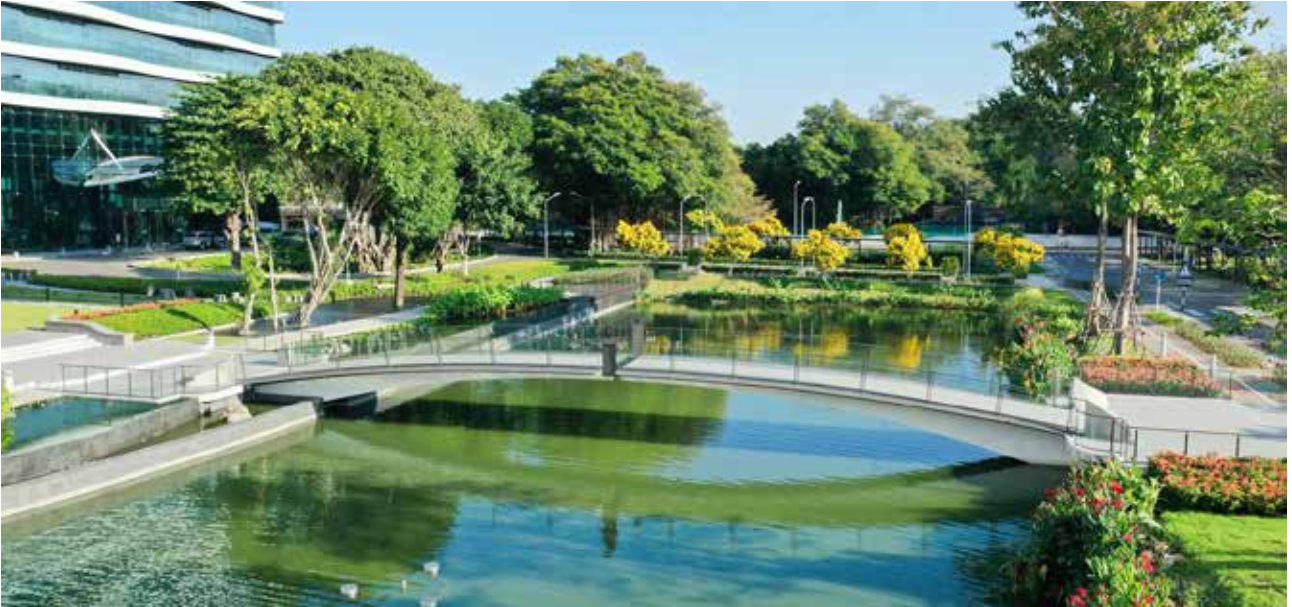
CPAC Ultra Bridge Solution, the innovative, the first thinnest concrete bridge in Thailand and ASEAN with UHPC (Ultra-high Performance Concrete) technology
