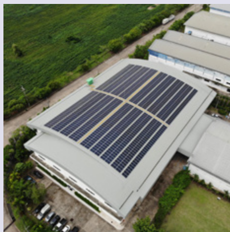
Photo of the 2nd solar power generation system; size 380 Kw, at Prachinburi branch factory
