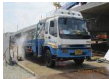
Photo depicting water spraying to reduce dust dispersion, speed limit for vehicles, and cleaning of wheels before leaving the construction site.
