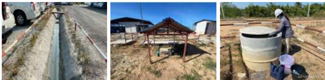
Photo depicting temporary water drainage ditches, temporary wastewater treatment system, and monitoring of wastewater quality in the project site
