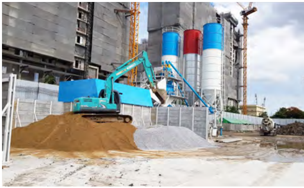
Set up Temporary Concrete Production Plant within the Project Reduces Pollution Caused by Transportation and Traffic Congestion Outside the Project.
