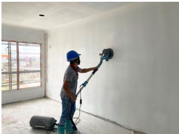
Use Vacuum Cleaner to Reduce Dust and Pollution Caused by Architectural Work
