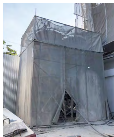
Use Plaster Silos and Plaster to Level the Floor to Reduce Pollution Caused by Transportation
