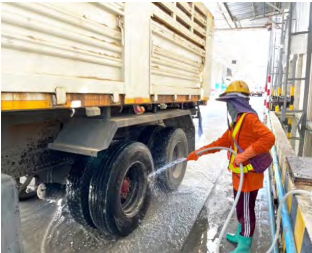
Wash Car Wheels to Prevent Leftover Soil from Getting onto the Road and Clean the Project Areas to Reduce Dust.
