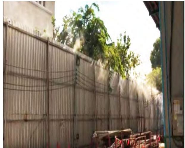
6 Meters High Fence with Water Sprayer Installed Temporarily Around the Project to Prevent Noise and Dust
