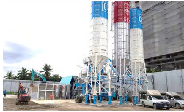
Set up Temporary Concrete Production Plant within the Project Reduces Pollution Caused by Transportation and Traffic Congestion Outside the Project.
