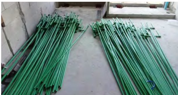
Assemble the finished pipe before installation to reduce pipe debris
