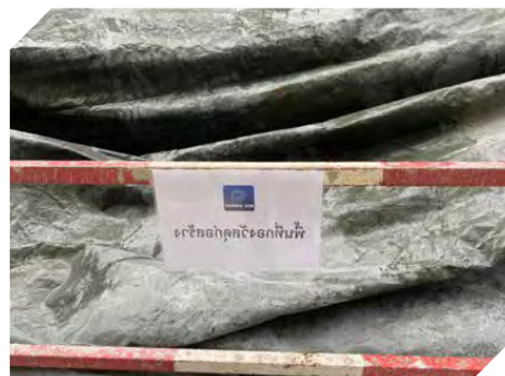
Cover construction materials with tarp to reduce dust within the project
