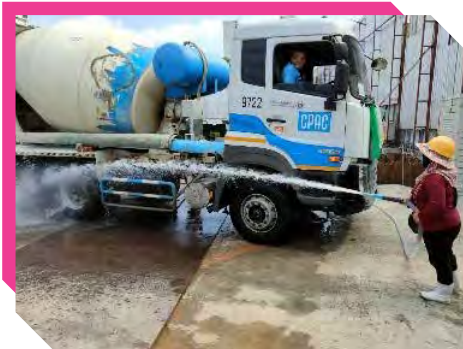
The wheels of vehicles entering the project are cleaned to prevent soil remnants on the road
