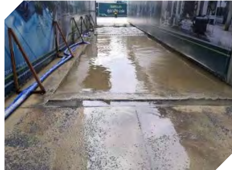
The wheels of vehicles entering the project are cleaned to prevent soil remnants on the road
