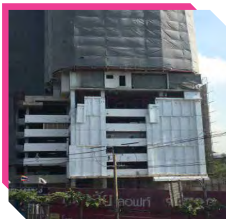
Precast walls are used instead of masonry walls to reduce environmental impacts
