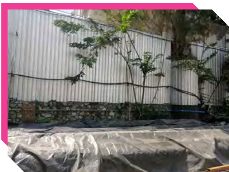
Cover construction materials with tarp to reduce dust within the project
