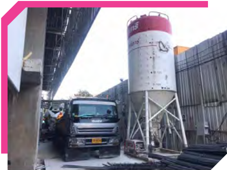
Plaster and floor concrete silos are used to reduce transportation pollution
