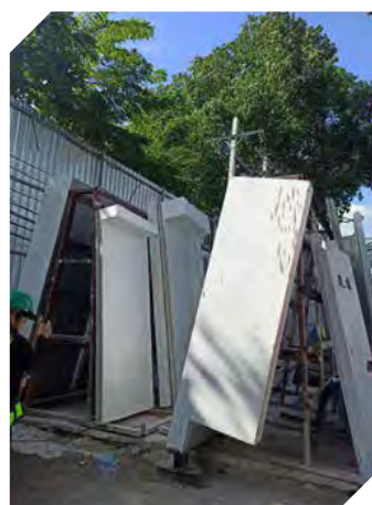
Precast walls are used instead of masonry walls to reduce environmental impacts
