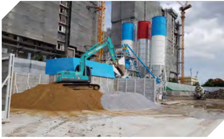
Temporary concrete plant is set up within the project to reduce transportation pollution
