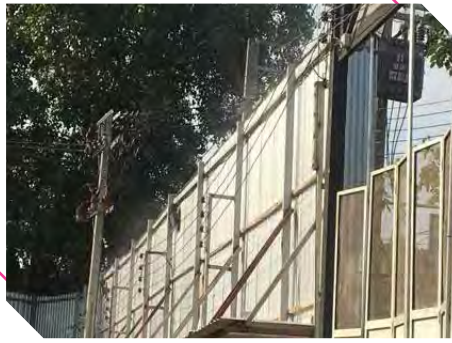
6 - meter high fence and installed water sprayers around the project to protect against sound and dust
