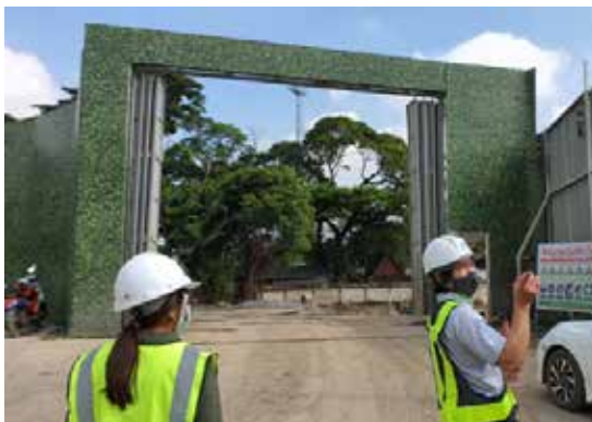
Image: installation of the solid fences around construction area
