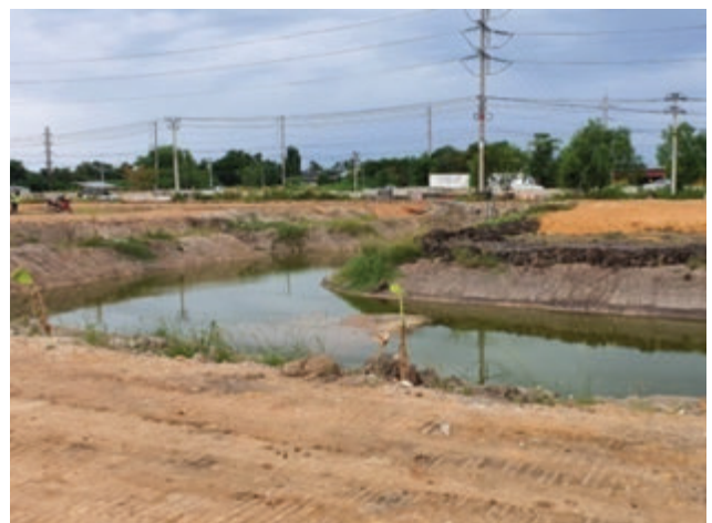
Image: drainage way and sedimentation tank
