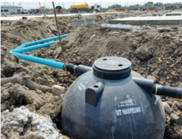
Image: installation of wastewater treatment tanks or concrete pond systems for wastewater treatment
