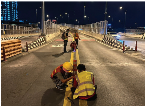
Image: The traffic poles installation at Khlong Noi Bridge
