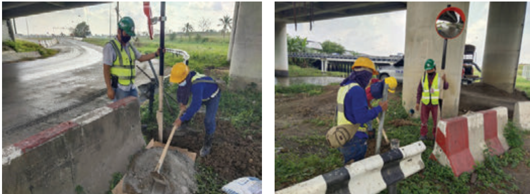
Image: Installing a convex mirror at the blind spot at the project's exit point
