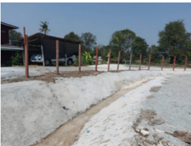
Image: drainage way and sedimentation tank
