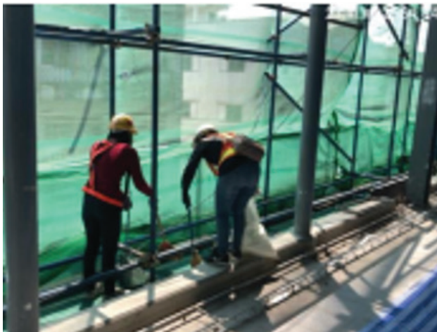
Image: installation of safety net to catch construction materials from high-level work
