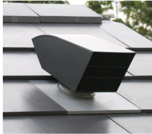
Passive Ventilation system, which is cooled under the roof with natural wind, Noble Gable Watcharapol Project
