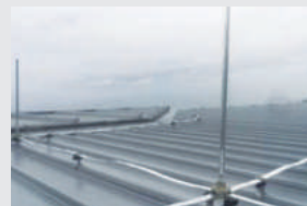
Installation of Lightning Protection at Min Buri Market Station (PK29)
