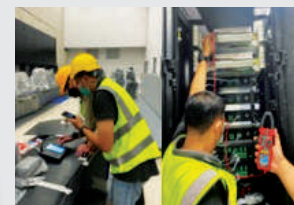
Subsystem stand-alone test (SSAT) for Public Announcement communication system at OCC Building
