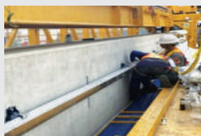
Installation of Conductor Rail between Srinakarin 38 Station (YL14) and Suan Luang Ror 9 Station (YL15)
