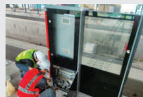
Installation of station doorways
