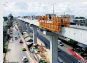
Installation of conductor rail near Setthabutbampnen Station (PK28) and Min Buri Market Station (PK29)
