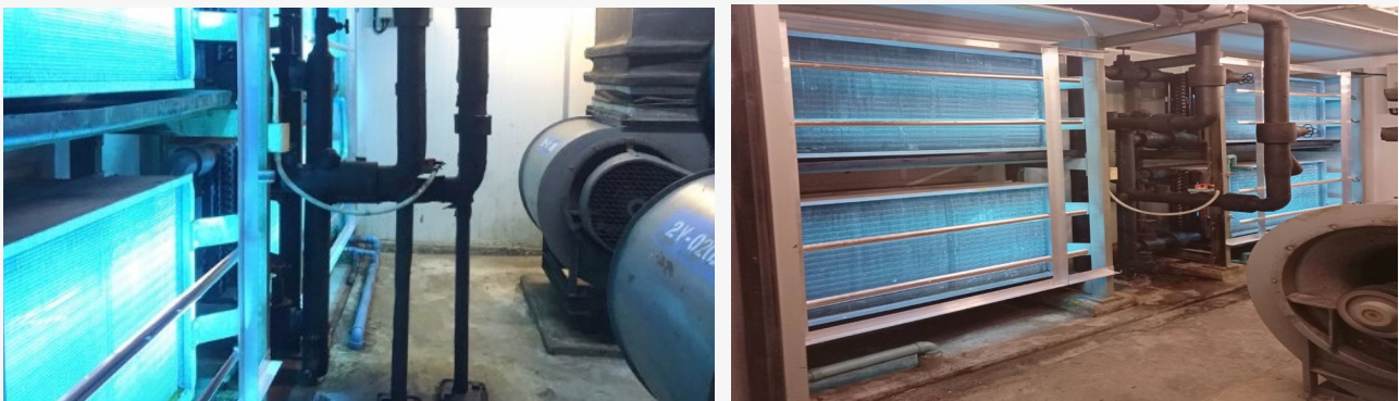
Install a UVC System to Sanitize Air Conditioning System
