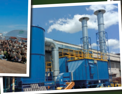
Installed the wet scrubber system for Concrete tile production line - CT4
