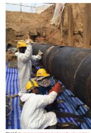
Figure 5. By moving an induction head over the pipe coating, the surface is instantly heated to 140 - 150°C before the coating is easily scraped off by using scrapers.
