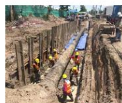
Figure 2. After excavation, the trench walls are secured and the ground under the pipe is covered by a concrete to offset debris from the removal process. Prior to starting the inductance removal process, the pipe is cleaned from dirt and gravel.
