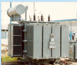
Open type conservator tank
