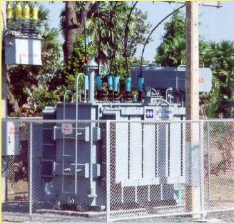
Open type conservator tank
