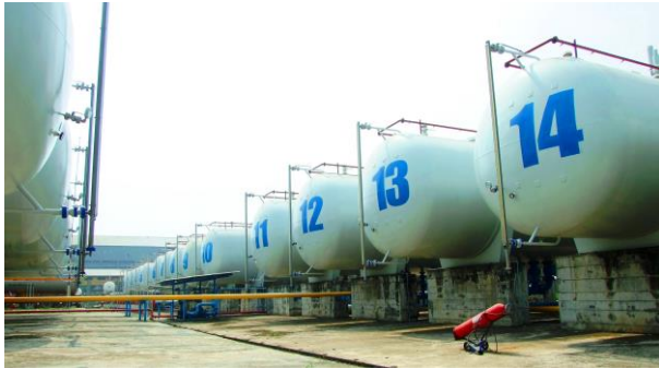
ถังเก็บก๊าซ LPG (BULLET TANK)
