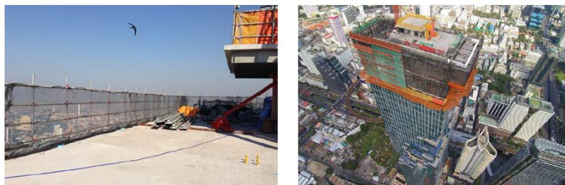
The use of skeletal mesh panels for prevention of falling materials around MahaNakhon Tower.
