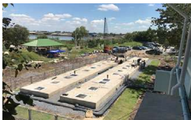
Installation of waste water treatment from hospital: before releasing into the natural water resources
