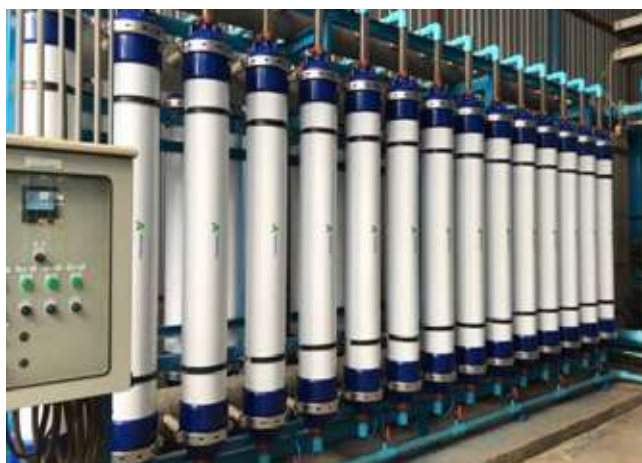
Installation of UF Membrane for water treatment
