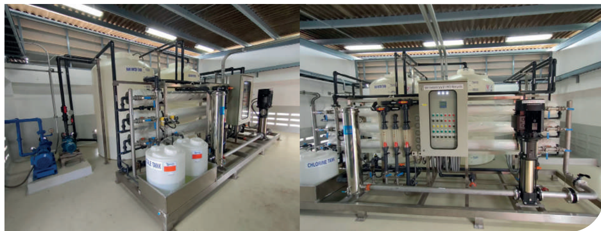
UVLA 3200-8 (2 sets) 150 m3hr. installation project (ThaiNamthip Limited, Factory in Nakhon Ratchasima Province)
