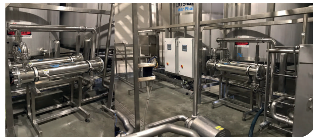
Improvement system for wastewater treatment system and overload protection (ThaiNamthip Limited, Factory in Nakhon Ratchasima Province)
