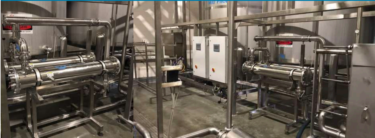
UV Guard model X4-440 installation project (ThaiNamthip Limited, Factory in Rangsit-Pathumthani)
