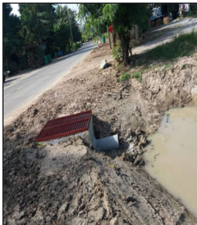
The Project to embed drainage pipe with manhole at village no.7 Baan Sa Bua Kam, distance 138 Metres at a budget of Baht 339,000, for preventing the flood. This project is a part of Cooperation for Community Development Social and environmental sustainability project.
