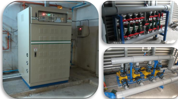
Ozone for Cooling Tower, ESPLANADE
