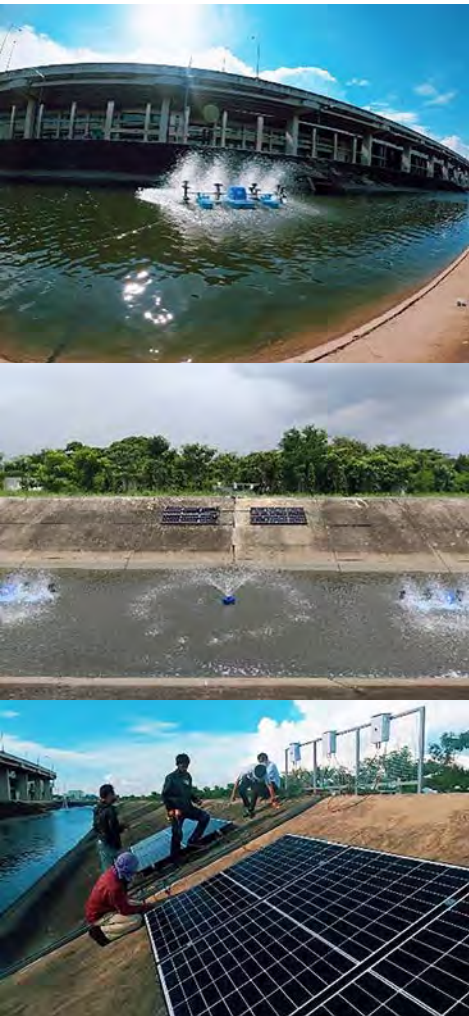
Generation of electricity from solar energy for water treatment in natural canals
