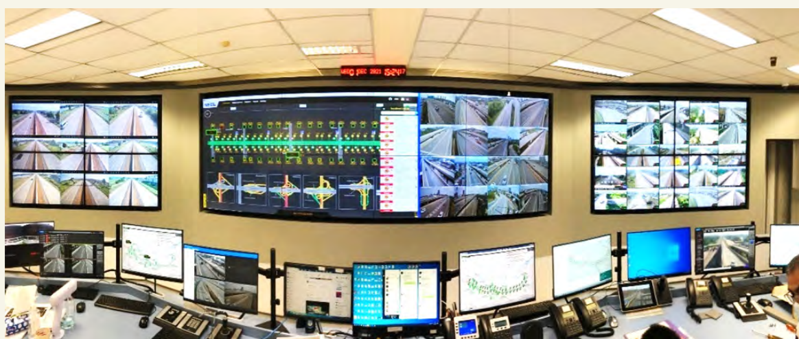
Intelligent Video Analytic (IVA) and Alert at Udon Rattaya Expressway Control Center
