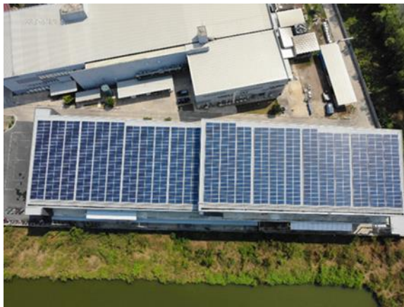
Solar power generation system (Solar Rooftop) on the roof of the new factory building
