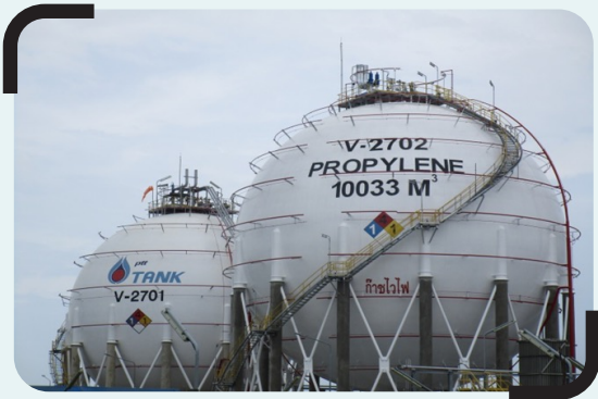
Project : PTT Tank Terminal Propylene Spherical Tank Propylene Storage 4,000 tons.
