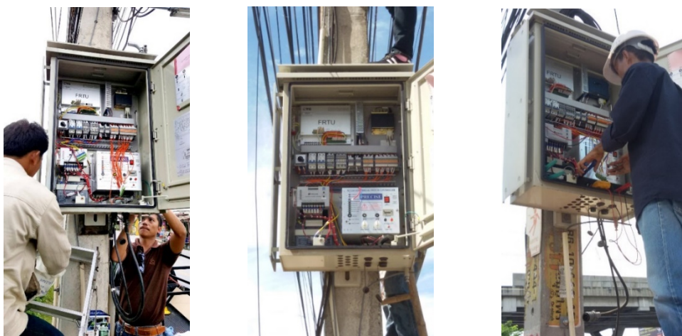
FRTU System Installation
