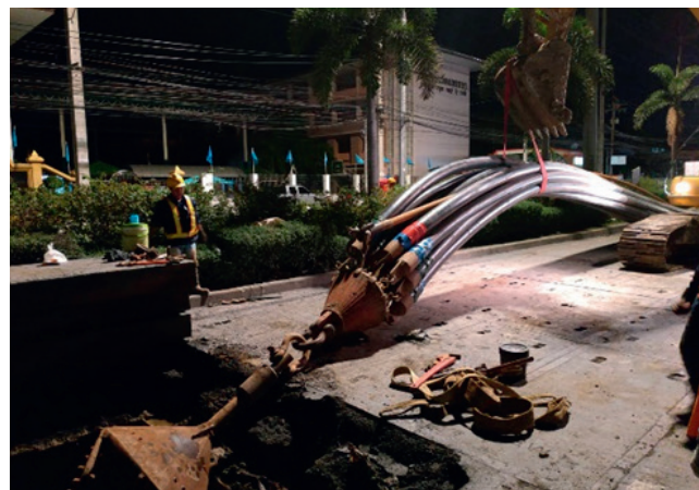
Pipe Jacking & Manhole, Yellow Line MRTA Project, Bangkok (Horizontal Directional Drilling Method)
