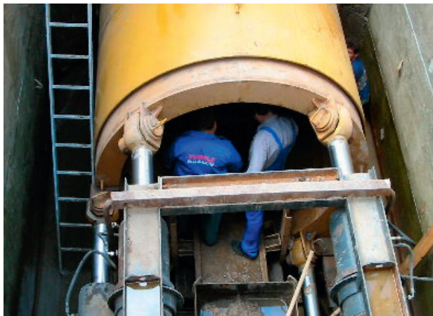
Pipe Jacking & Manhole, Prag - Gasa Station Project, Samut Prakan
