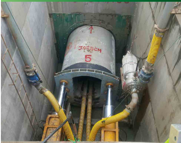
Pipe Jacking & Manhole, Prag-Gasa Station Project, Samut Prakan, Thailand
