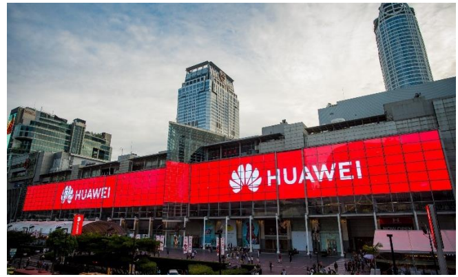
CentralWorld (ongoing renovation)
