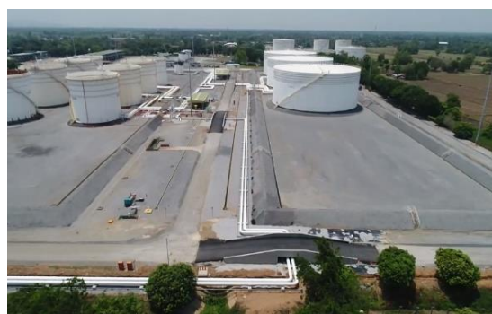
The Extension of the Petroleum Pipeline System to the Northeastern Region Project (TPN)
